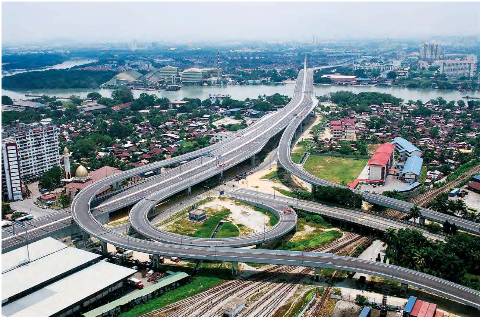
The Butterworth Outer Ring Road in Penang was constructed to serve the metropolitan areas of Butterworth and Bukit Mertajam that have seen a surge in vehicular traffic with intense industrial and urban development. The 14-kilometre expressway has six elevated interchanges and a bridge over Sungei Perai.
