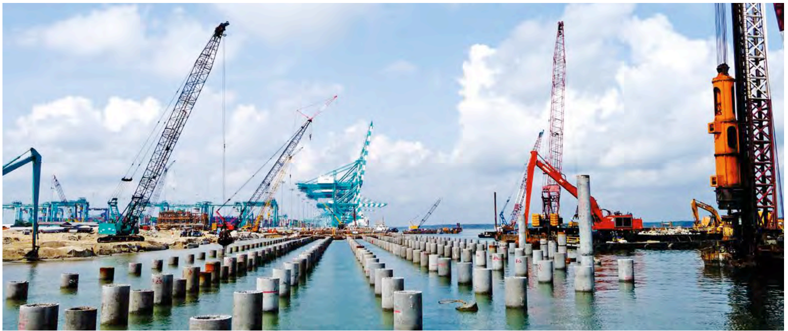
ICP piles were used in Berths 11 and 12 of Port of Tanjung Pelepas in Iskandar Malaysia.
