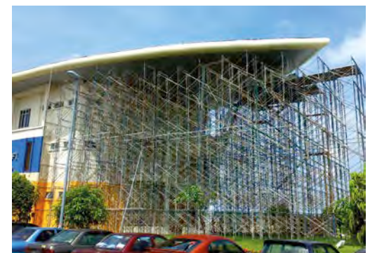
IJM provided the scaffolding during roofing and ceiling works at the Tentera Laut DiRaja Malaysia training facility.
