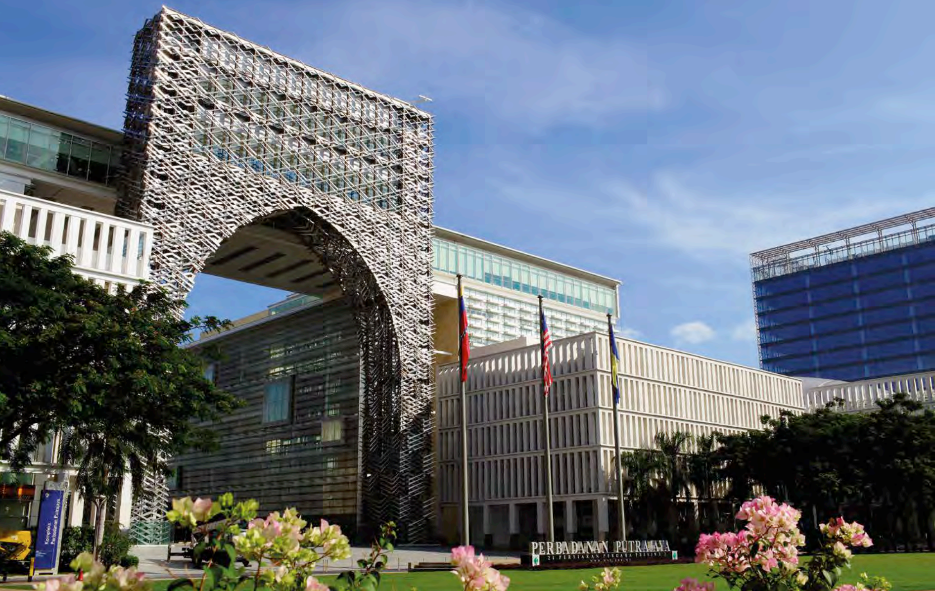
IJM built the steel-clad façade of the head office of Putrajaya Corporation.
